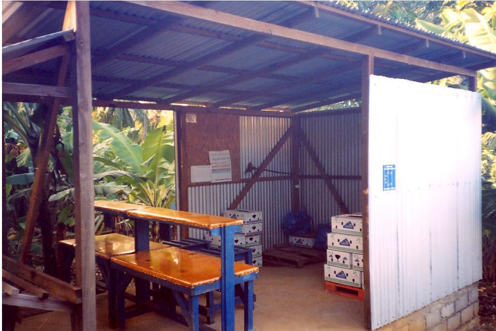
Figure 12: Simple field shed
