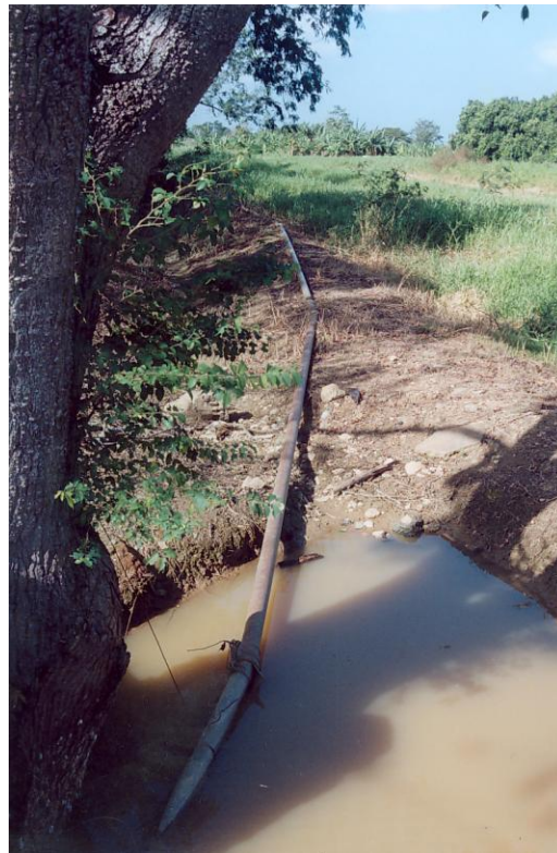
Figure 9: Galvanise conduit with pumping polluted water into production fields
